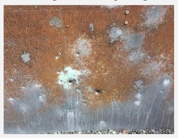
This a picture of the plate designed to protect the trap house from being hit by incidental birdshot. This is not a target for testing slugs. This deliberate damage is uncalled for and causes range funds to be diverted to needless repairs instead of regular maintenance or expansion.
